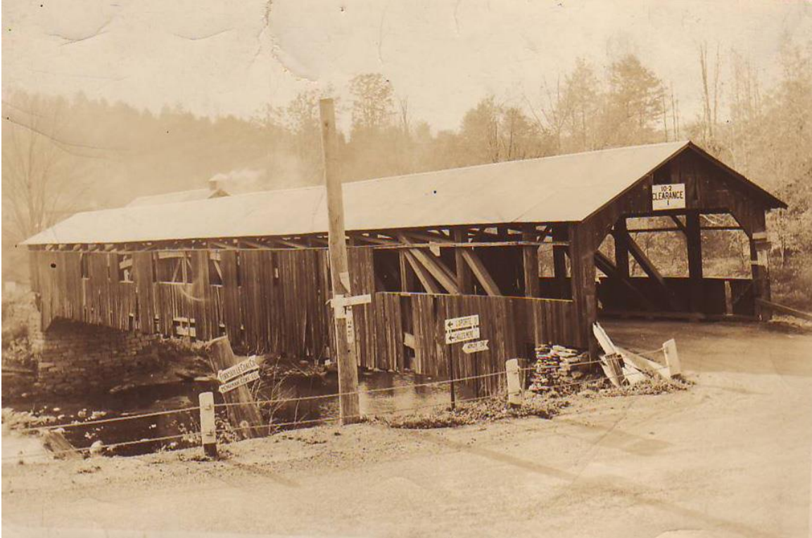
Forksville covered bridge
